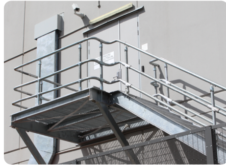
INDUSTRIAL STAIRCASE HANDRAIL
