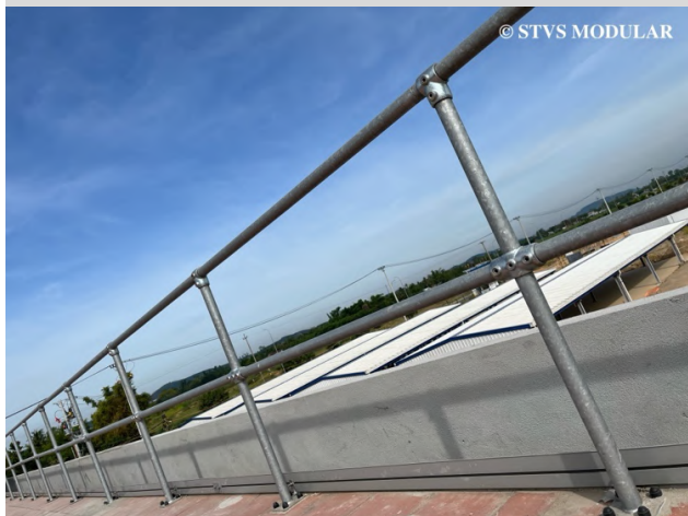
ROOF HANDRAIL
